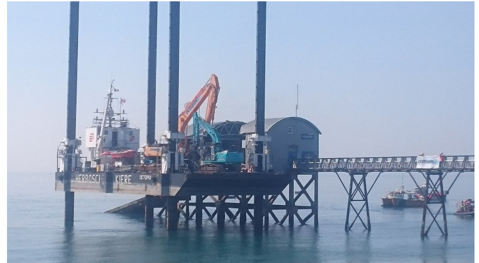
Demolition of Selsey Lifeboat Station
